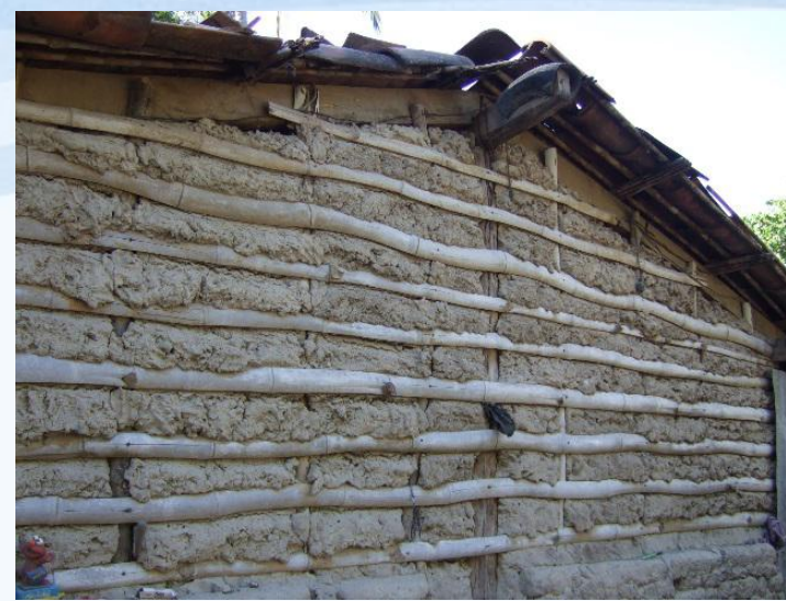
Traditional rural Bahareque housing in El Salvador. No outer render has been applied (It is known as wattle-daub in UK)
